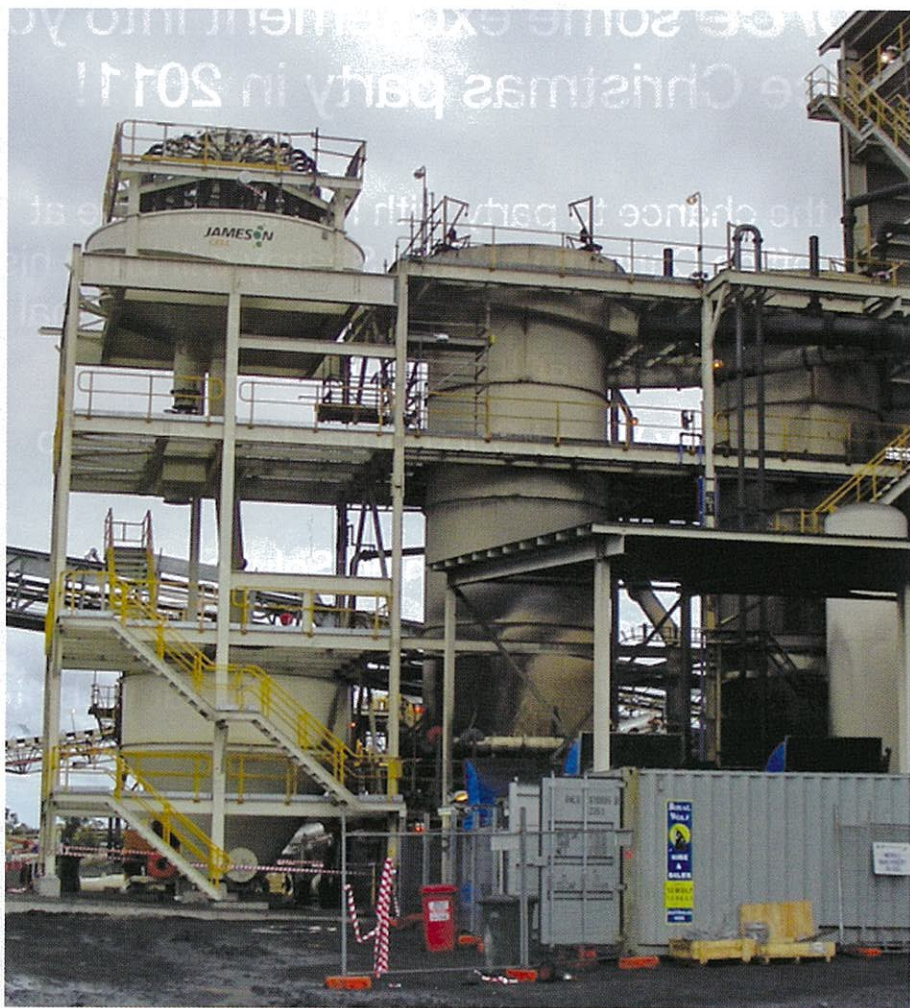
The Jameson Cell being installed at Anglo American's Lake Lindsay CHPP.
